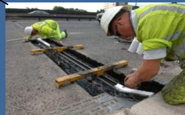
USL - Bridge Expansion Joints
