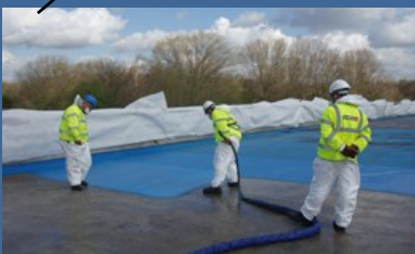
PmB - Polyurethane Waterproofing system
